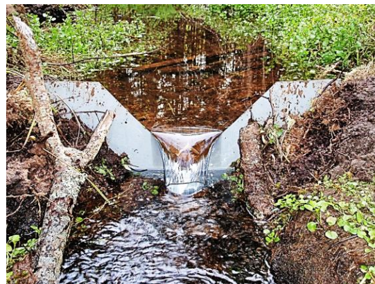
Figure 7-21. V-Notch Weir
