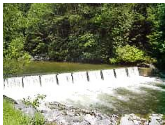
Figure 7-22. Rectangular Notch Weir
