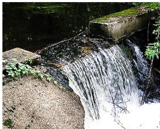
Figure 7-24. Broad Crested Weir
