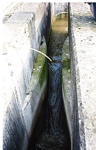
Figure 7-26. Venturi Flume
