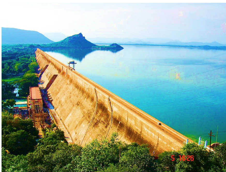
Figure B-3: 1700 m long Masonry Gravity Dam
