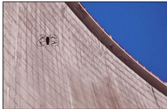
Figure 8-4. An inspection drone at work photographing the downstream face of the Tseuier Dam in Valais, Switzerland
