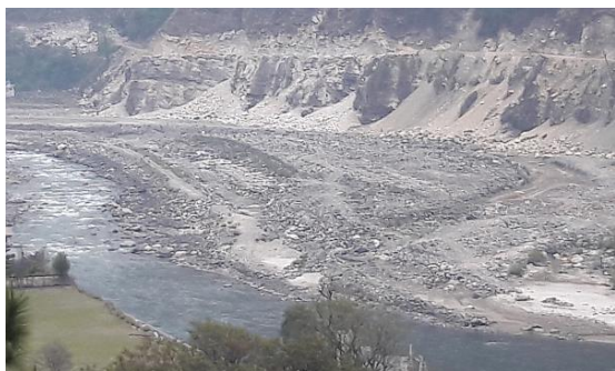
Figure 6-30. Large amount of sediment, inflowing in to the upstream reach during road construction
