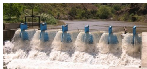
Figure 4-43. The Fusegates in Black Rock Dam, US (upper) and Vorotna Dam, Armenia (lower) ( www.hydroplus.com )
