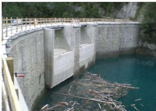
Upstream of dam
