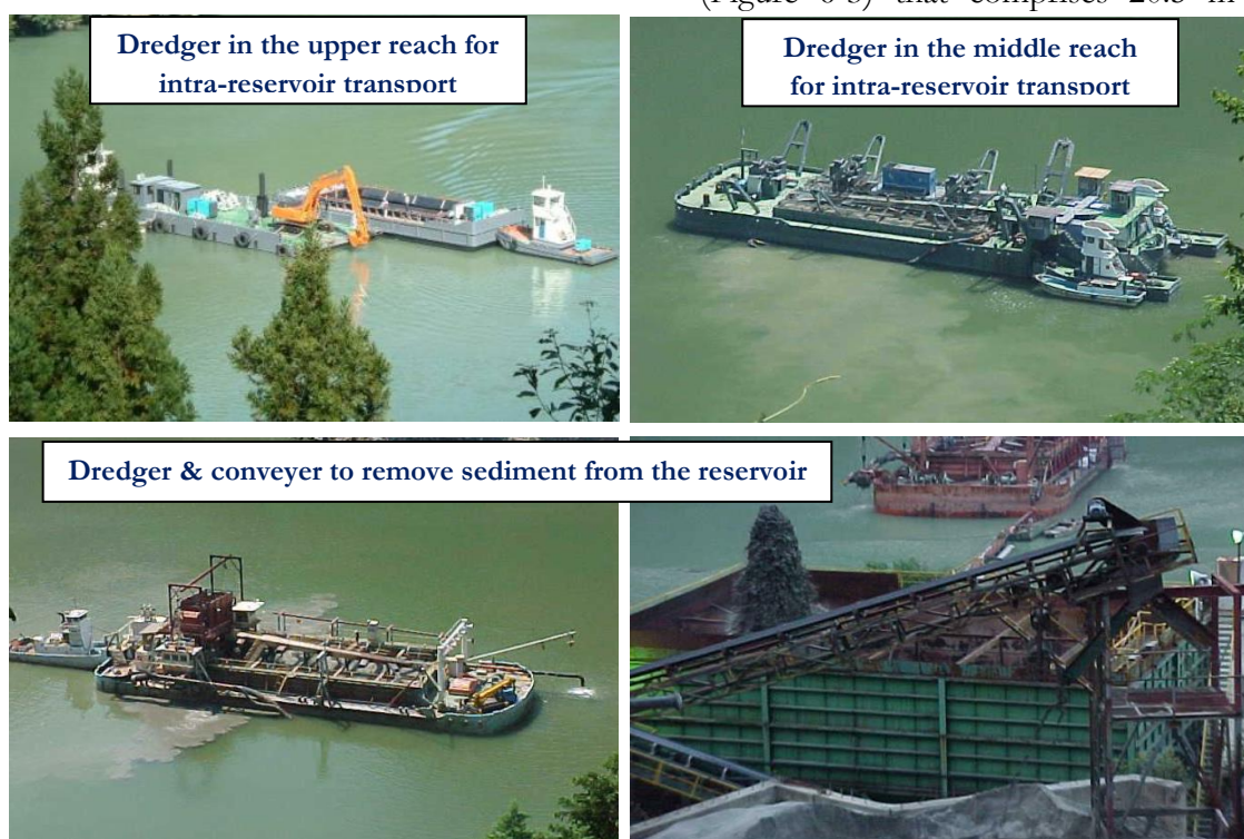
Figure 6-2. Sediment dredging and removal arrangement ( J-Power, personal communication )
