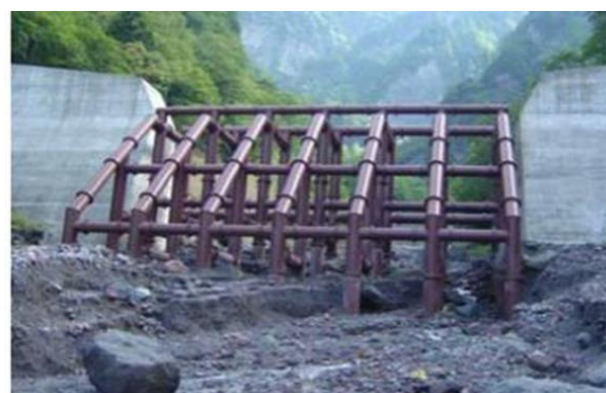
Figure 4-5. Sabo/check dam from steel pipes (Sumi and Kantoush, 2010)
