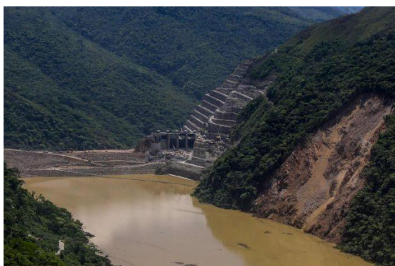
Figure 3-3. Shallow landslides at Hidrotuango reservoir in Colombia ( Internet source )
