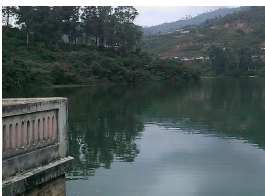
Figure 3-15. Kundah Palam reservoir during monsoon (upper picture) and low flow period (lower picture)
