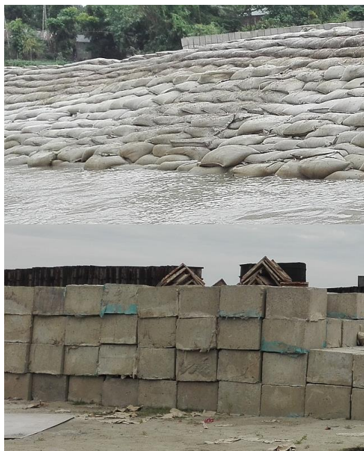
Figure 4-54. Bank protection in Brahmaputra (Bangladesh) using geo-bags and blocks (as products of dredged sand)
