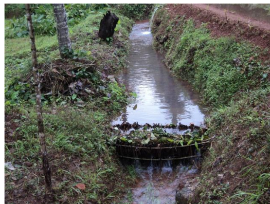
Figure 4-9. Brushwood check dam (Image: CRD, Kerala)
