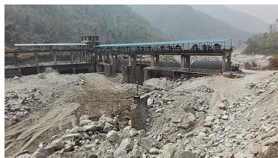
Figure 4-62. Sediment accumulation in a hilly HPP in Nepal ( Picture: S. Giri )
