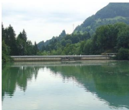
Upstream of dam
