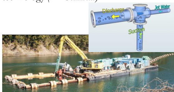
Figure 4-36. A EPDS installation in a Japanese reservoir ( Temmyu et al., 2013 )
