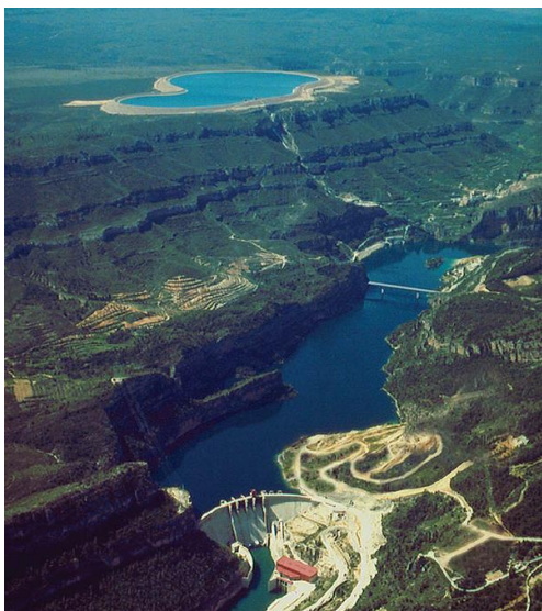
Figure 4-45. La Muela HPP with an additional pump storage pond ( Wikipedia )
