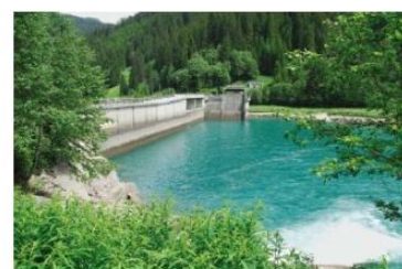
Upstream of dam
