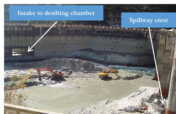
Figure 6-34. Sediment deposition in front of the spillway and the intake
