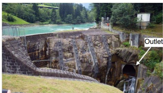
Downstream side of dam
