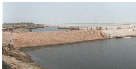
Figure 4-58. Sand plug with brick cover in Jamuna near Katlamari ( E. Mosselman, personal communication )
