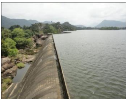
Figure 4-38. Spillway raise in Papanasam forebay in Tamil Nadu, India
