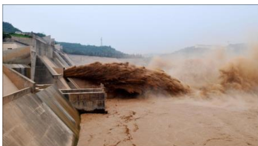
Figure 4-18. Sluicing of sediment-laden flow in the Xiaolangdi Reservoir on the Yellow River during a flood peak adjustment
