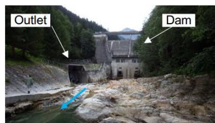
Downstream of dam
