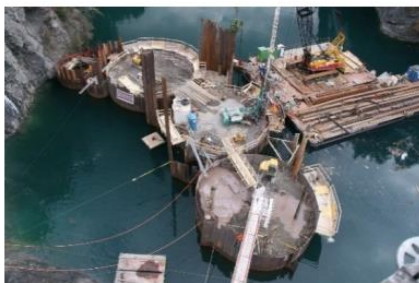
Circular-cell cofferdam (under construction)
