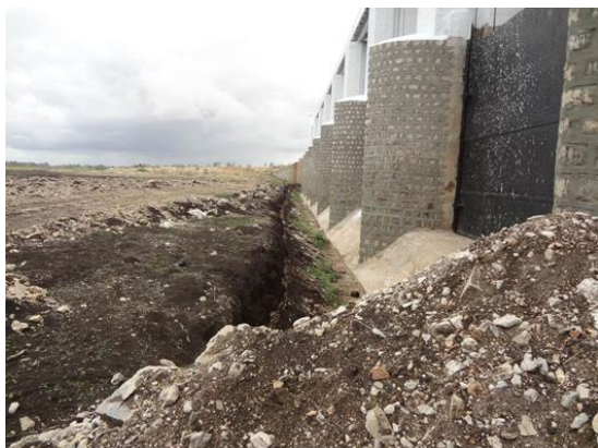
Figure 2-1. Deposition up to crest level, seen in an empty Hagari Bommanahalli reservoir in Karnataka, India
