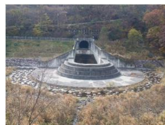
Tunnel outlet and energy dissipator
