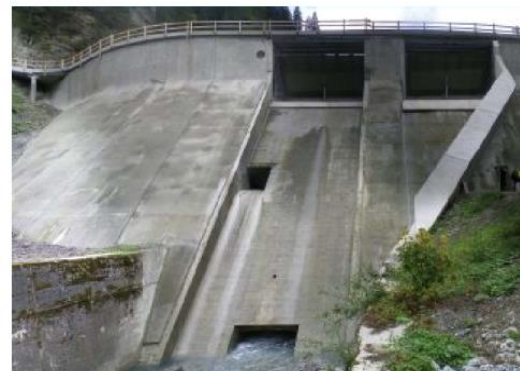
Downstream of dam
