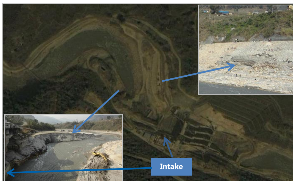
Figure 4-65. A Google earth image of dry Middle Marsyangdi reservoir with pictures of inner bend deposition near the intake and toe erosion at outer bend protection near the spillway
