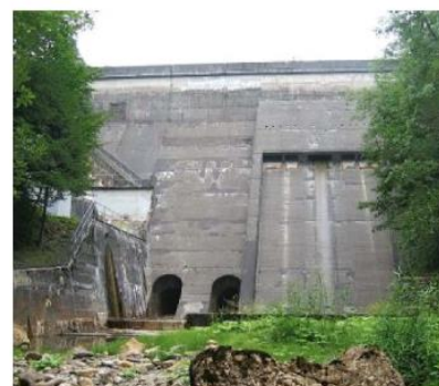
Downstream of dam
