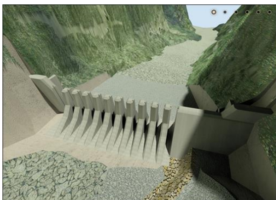
Figure 4-7. Slit dam in a hilly streams in Portugal, designed for a debris flow Q = 200 \text{ m}^3/\text{s} (Courtesy: LCW website)
