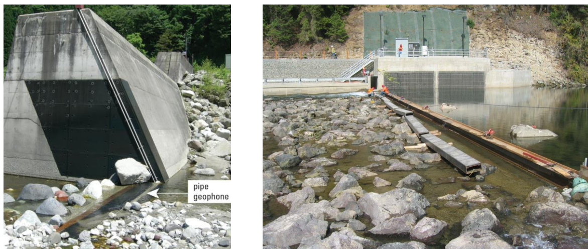
Figure A-1. Bedload measurement using pipe geophone (left), located on a stable bed surface of a slotted debris dam on the Joganzi River, Japan (Gray et al., 2010) and bedload impact plates and sensors, installed on the Elwha River, USA in 2009 (Hilldale, 2013)
