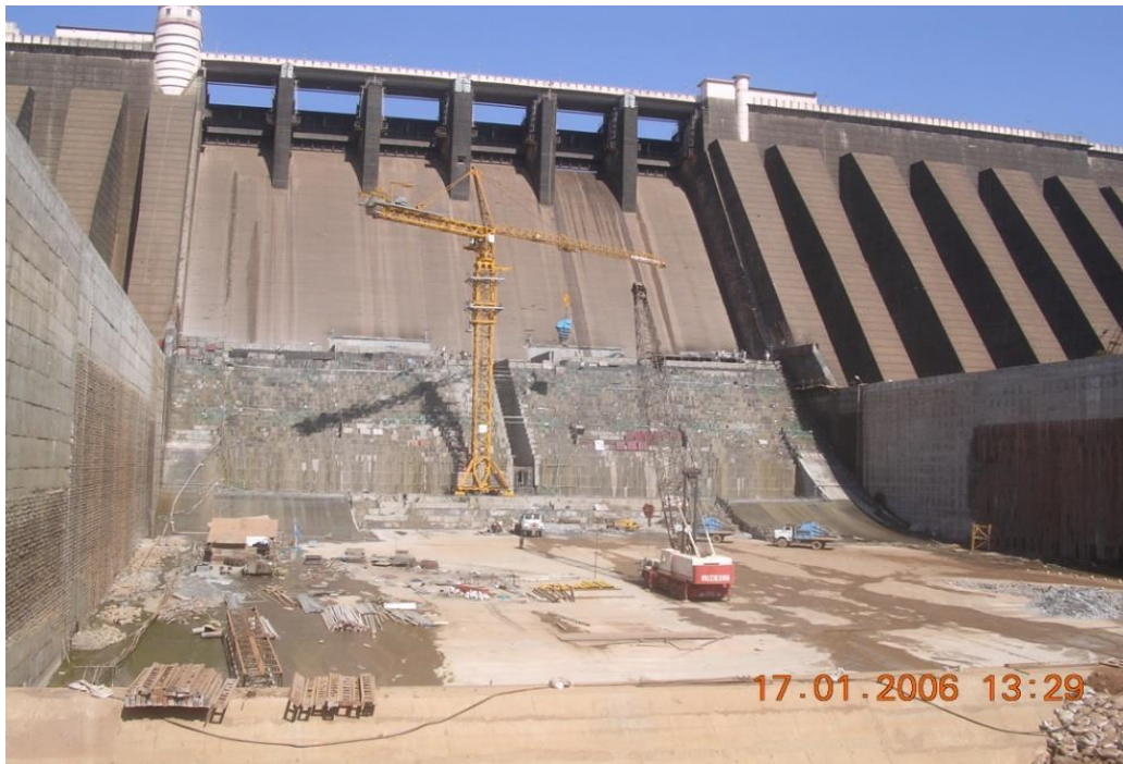
Figure 10: Photograph showing Second Year Strengthening work in progress
