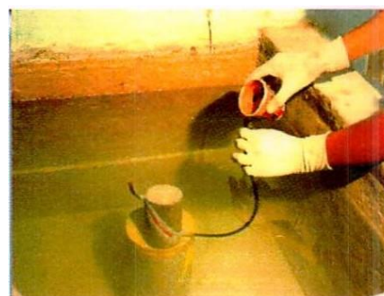
Figure 4-13: Underwater Grouting of Slant Cone
