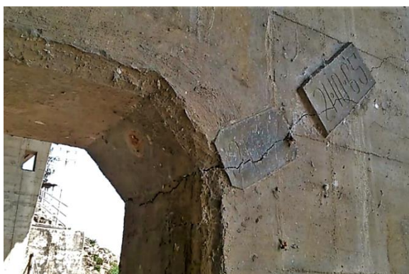
Photograph 7 - Cracks in downstream of Non-overflow section
