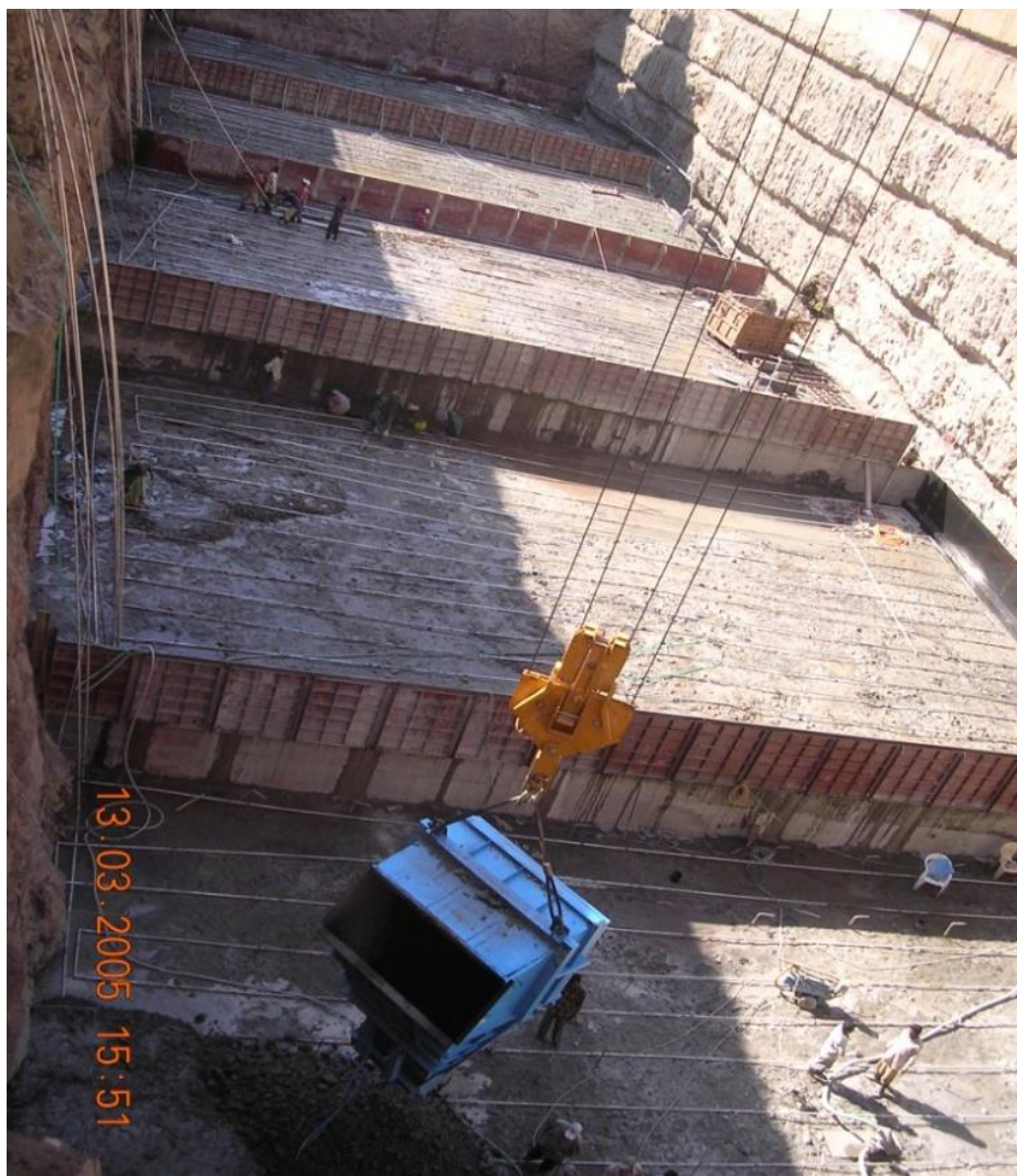
Figure 9: Photograph showing concrete placement and post cooling arrangement
