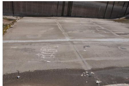
BLOCK 49 – PANEL C – AFTER EPOXY FINISH
