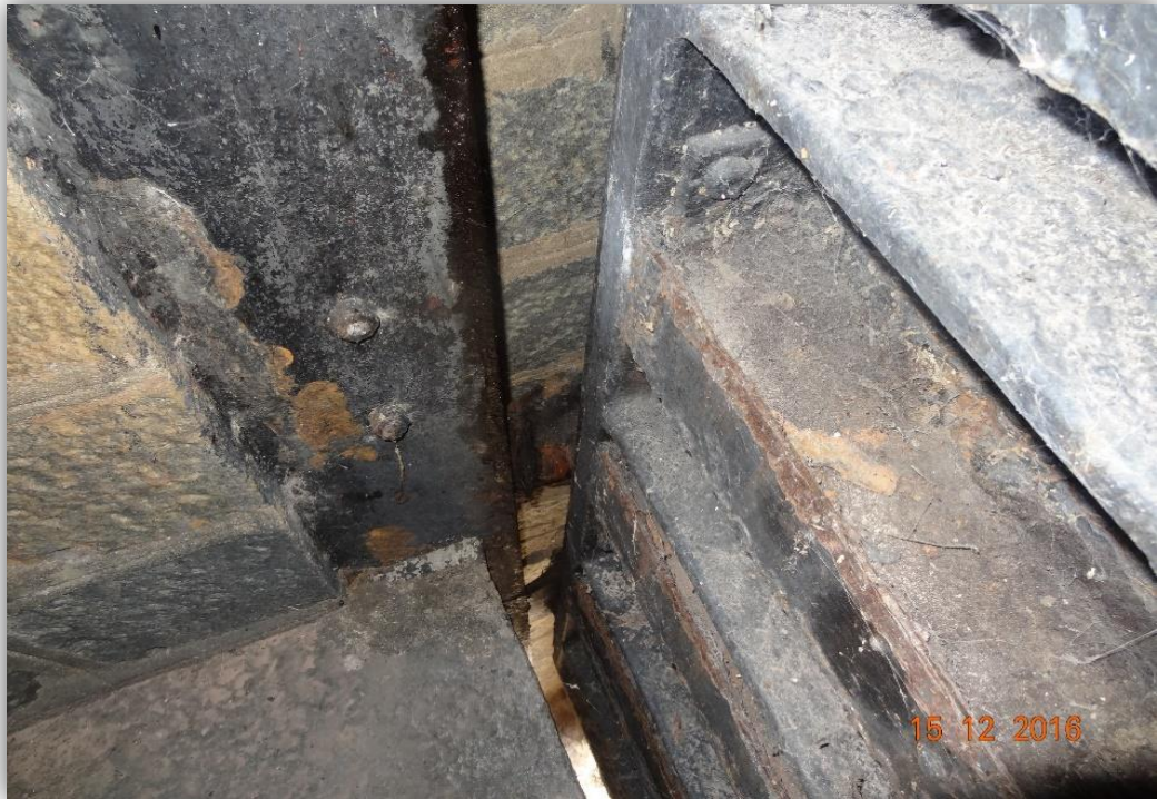
+103' gate and embedded parts - looking from d/s side.
