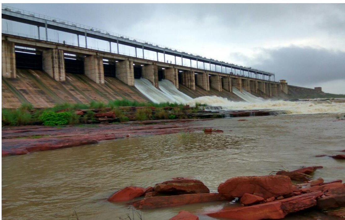
Figure 1 – Downstream view of Spillway
