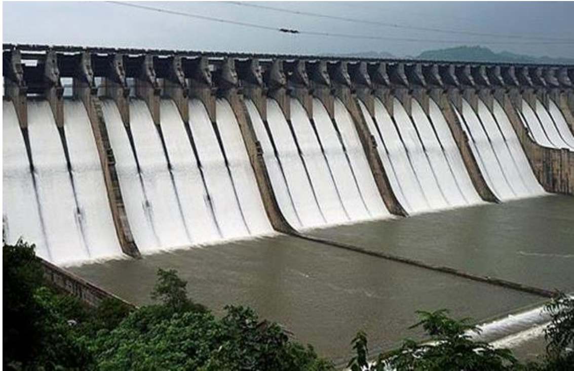
Downstream view showing the spillway
