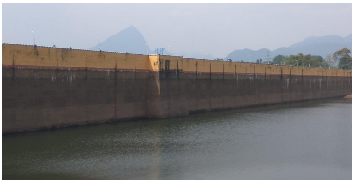
Figure 1(a) Upstream view of Pechiparai Dam
