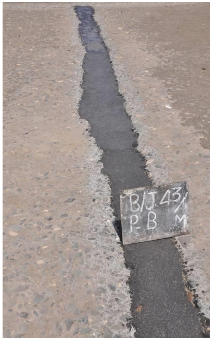
EPOXY TREATMENT IN JOINTS
