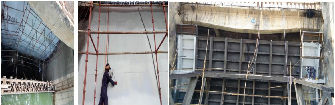
Spillway Gates Zinc Metallizing work at upstream side
