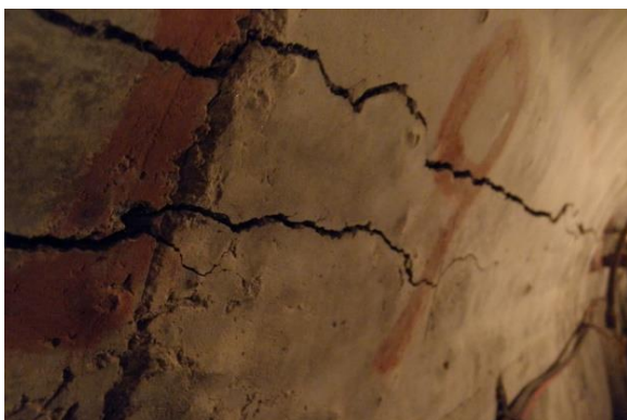
Photograph 3 - Entrance to hollow Spaces of the dam & Cracks in the Inspection gallery
