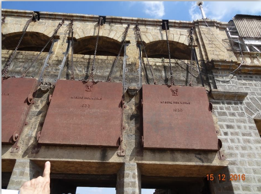
Existing +114' gates in hanging position over +103' sluices.
