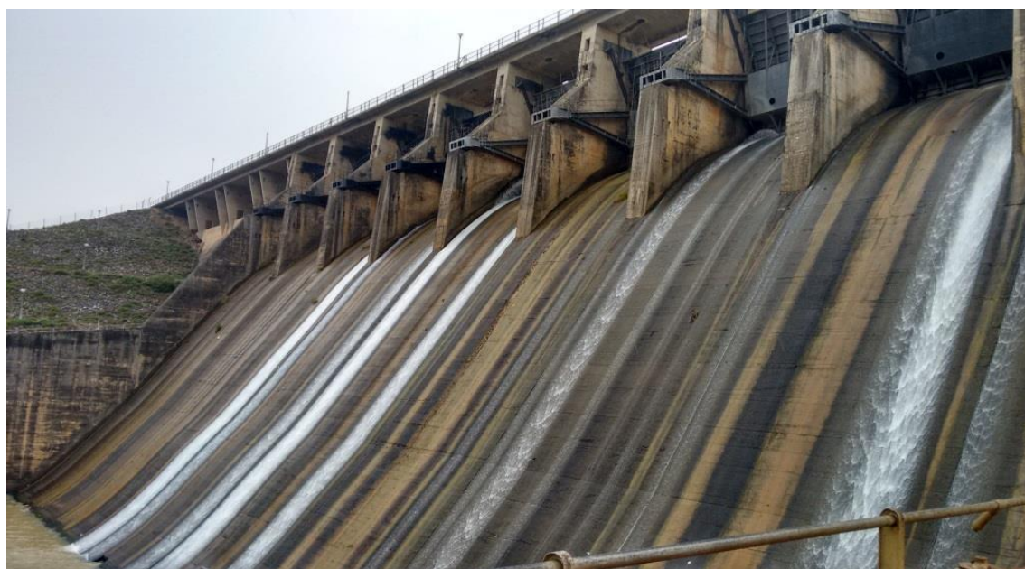
Figures 1, 2 and 3 show the Plan of Konar Concrete dam, downstream view and typical Non-Overflow and Overflow sections of the Concrete dam.
