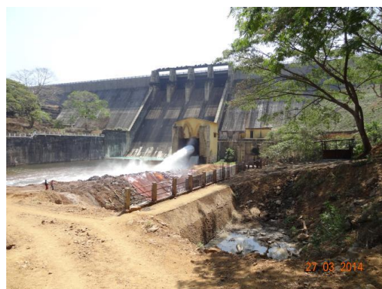
Figure - 2 Down Stream view of Masonry Spillway
