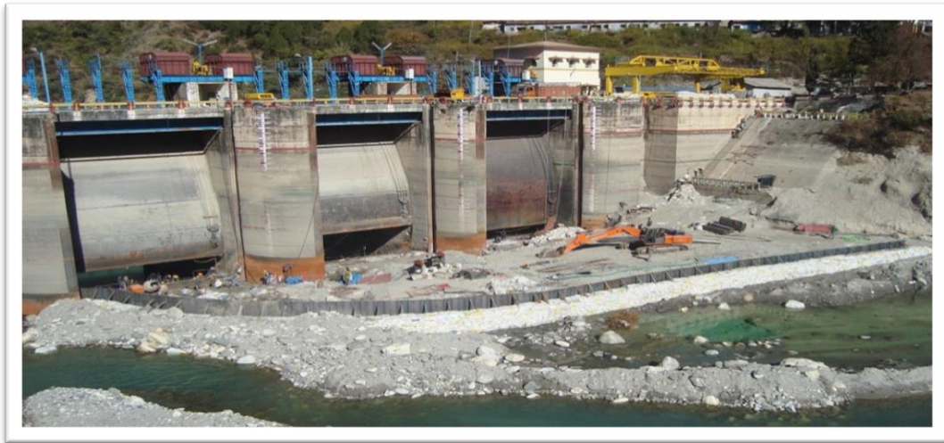
Photograph 2 (Temporary Bund for channelization of stream water)
