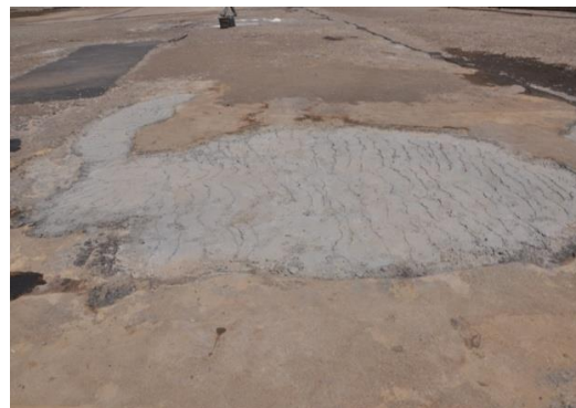
Bay-4 : BL. 44 – Panel-C – After Pouring Concrete
