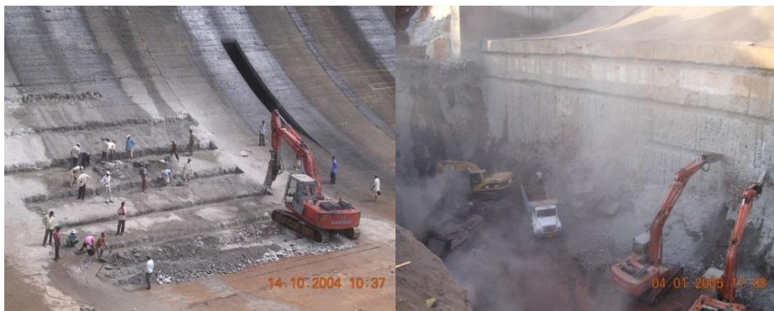
Figure 13: Cutting of Shear Keys
