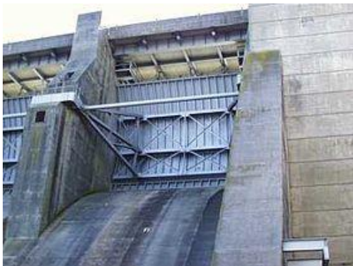
Figure 7-4: Spillway Radial Gates – Downstream Elevation
