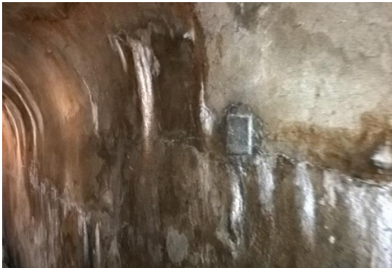
Photograph 5 - Cracks in Access/Operating gallery
