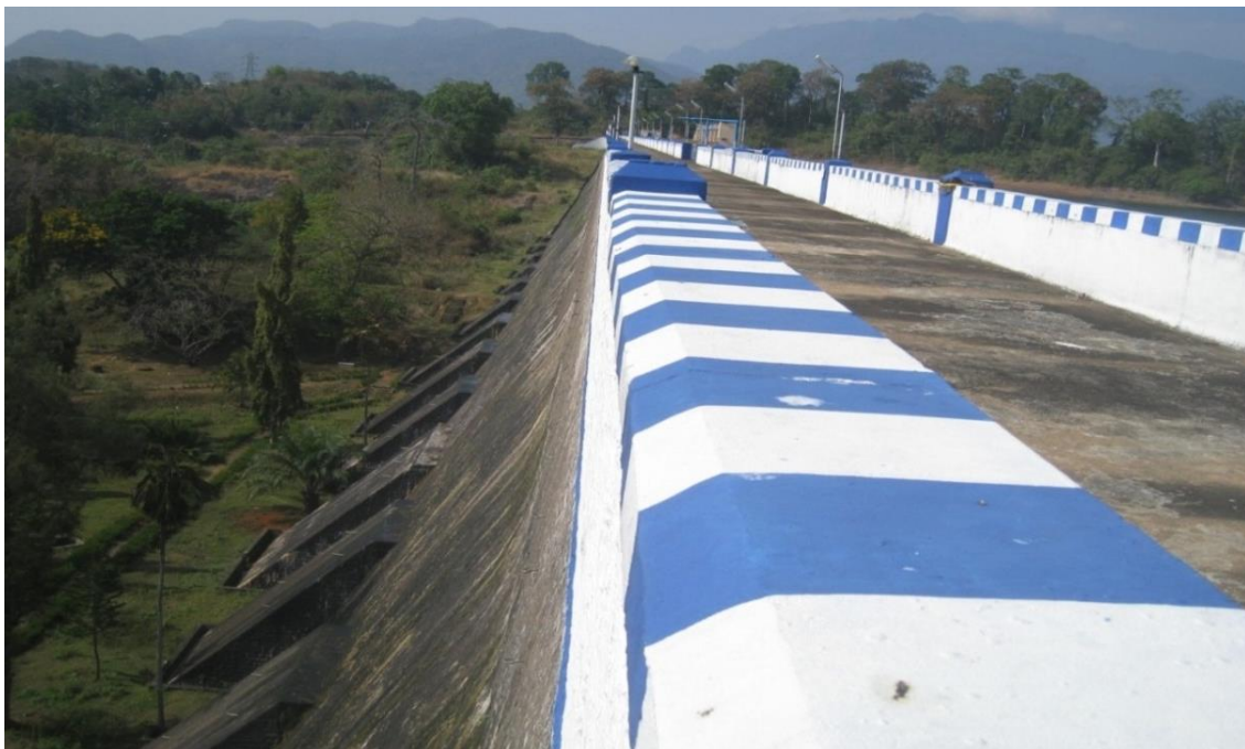
Downstream view of the existing dam with buttress
