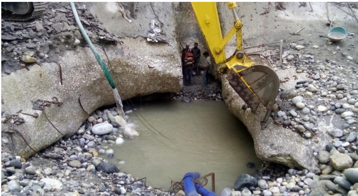
Photograph 6 (Cavity in Slotted Roller Bucket)
