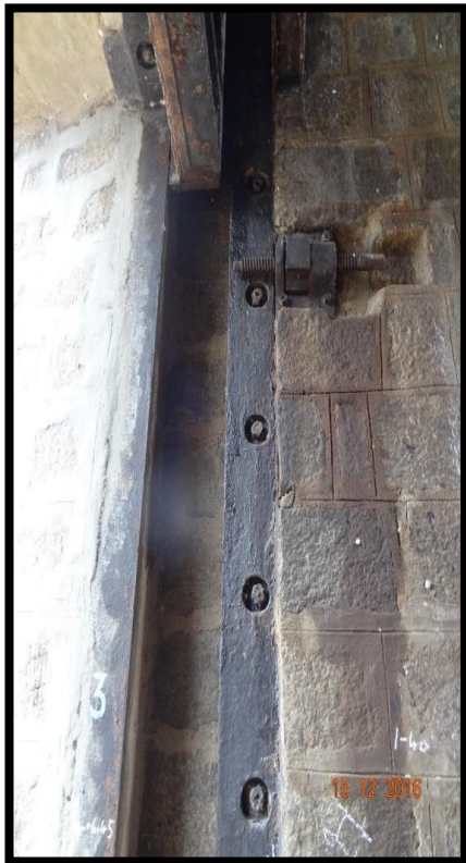
Existing gates groove and embedded parts for +106' gates
