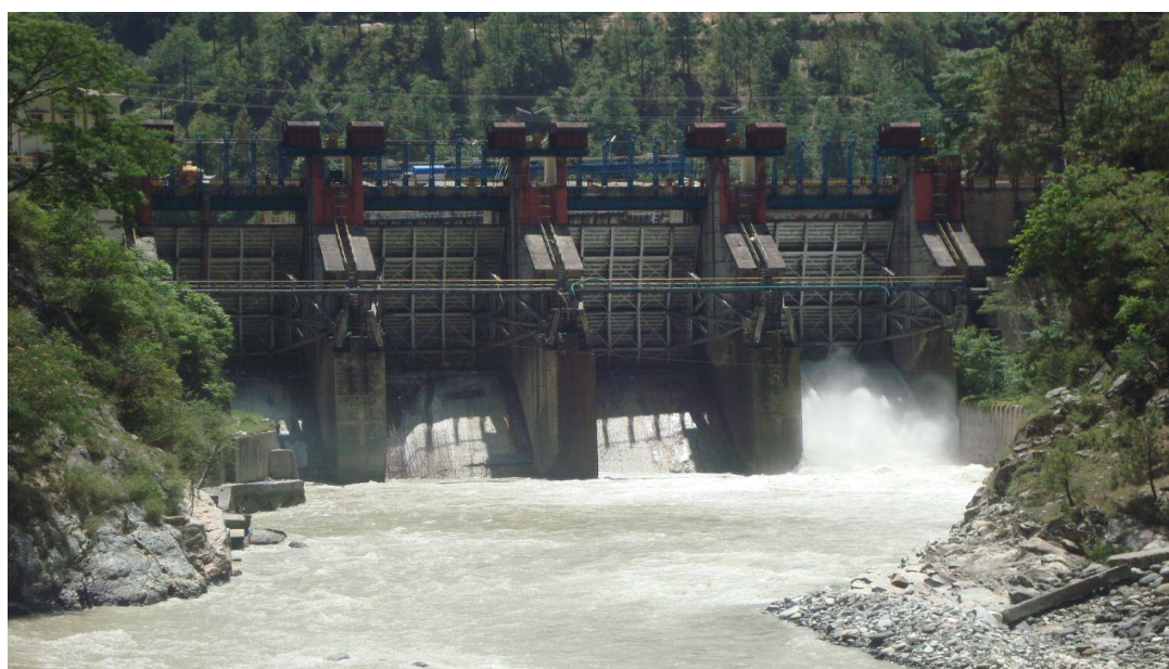
Downstream view of Maneri Dam
