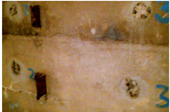
Photograph 6 - Cracks in Foundation/Drainage gallery
