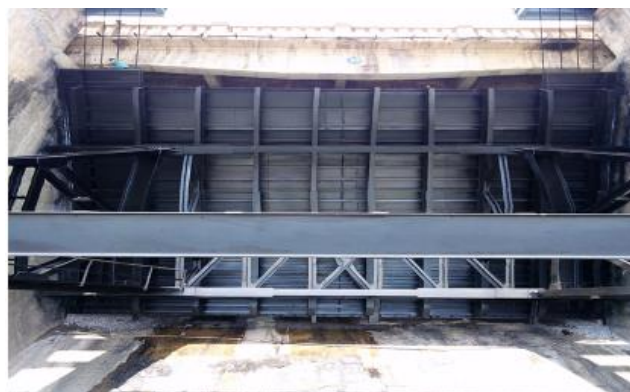
Painting to Spillway Gates
