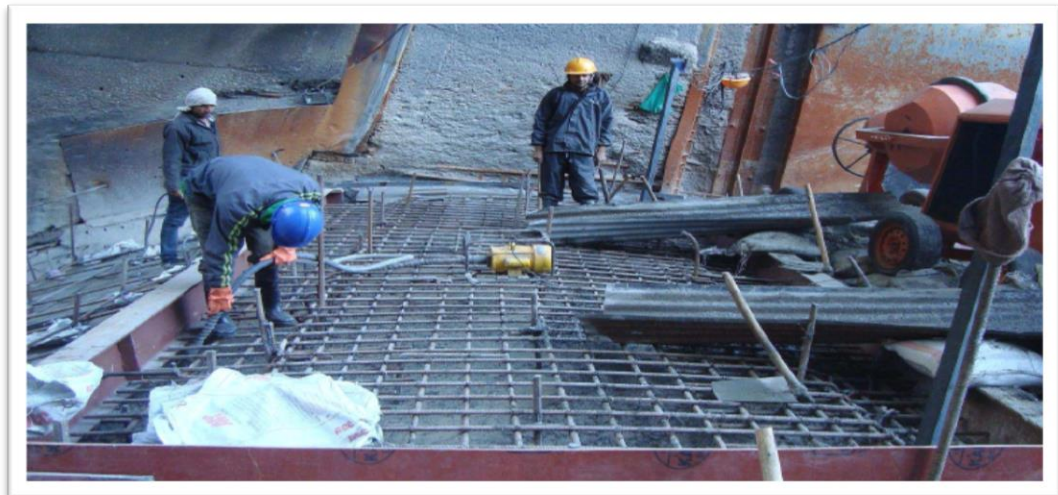
Photograph 3 (Laying concrete in spillway bay no 2)
