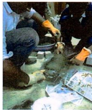
Figure 4-25: Repair Mortar Application on Specimen
