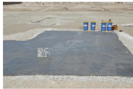
BLOCK 49 – PANEL C – AFTER EPOXY FINISH
