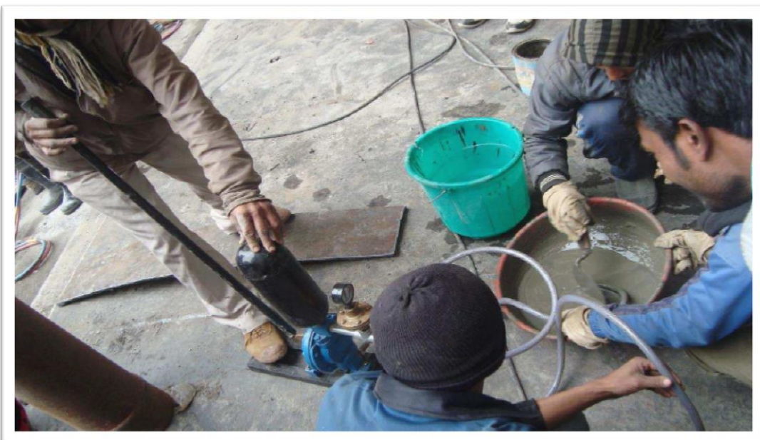
Photograph 4 (Laying and Grouting of MS Plate in Spillway bay no 2)
