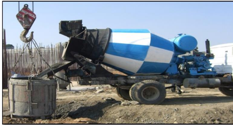
Photo 9: Delivery of concrete from transit mixer
