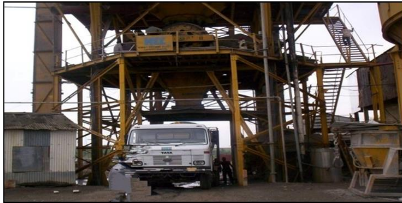
Photo 14: Mixture discharge into transit mixer
