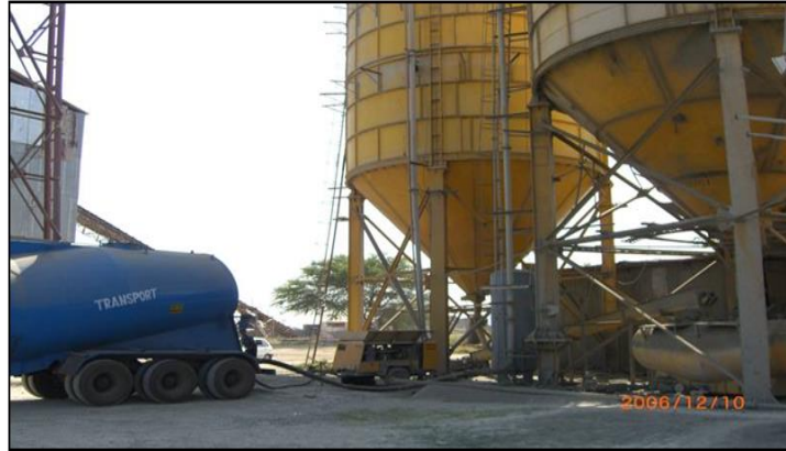
Photo 13: Cement silo-Cement feeding
