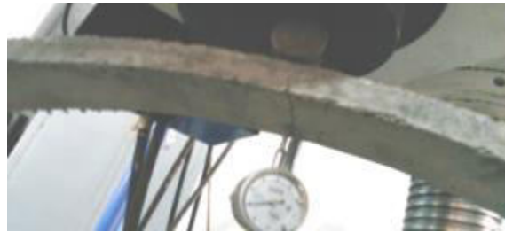
Figure 8. Crack on the bottom of arch
