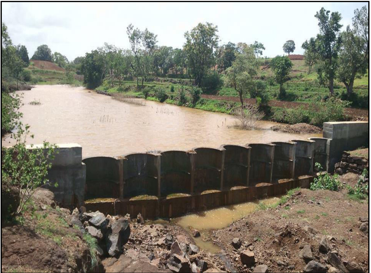
Ferrocement dam in Sakri, DistDhule.
