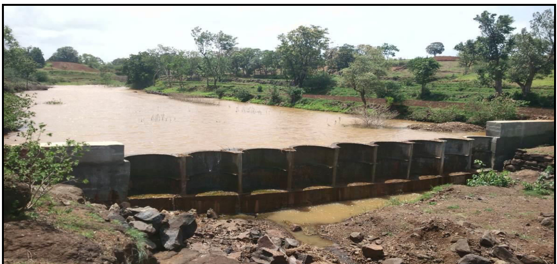
Fig 8.13 Bhandhara constructed with ferrocement at Dhule, India
