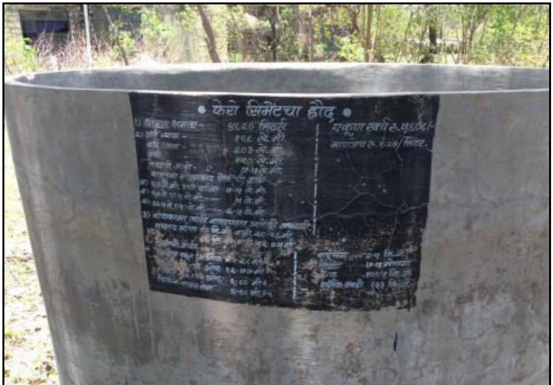
Water tank built in MERI Nashik in 1988
