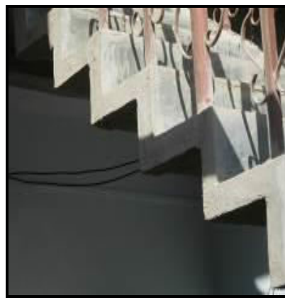
Fig 7.5 Steps using ferro-cement built near Katraj, Pune
