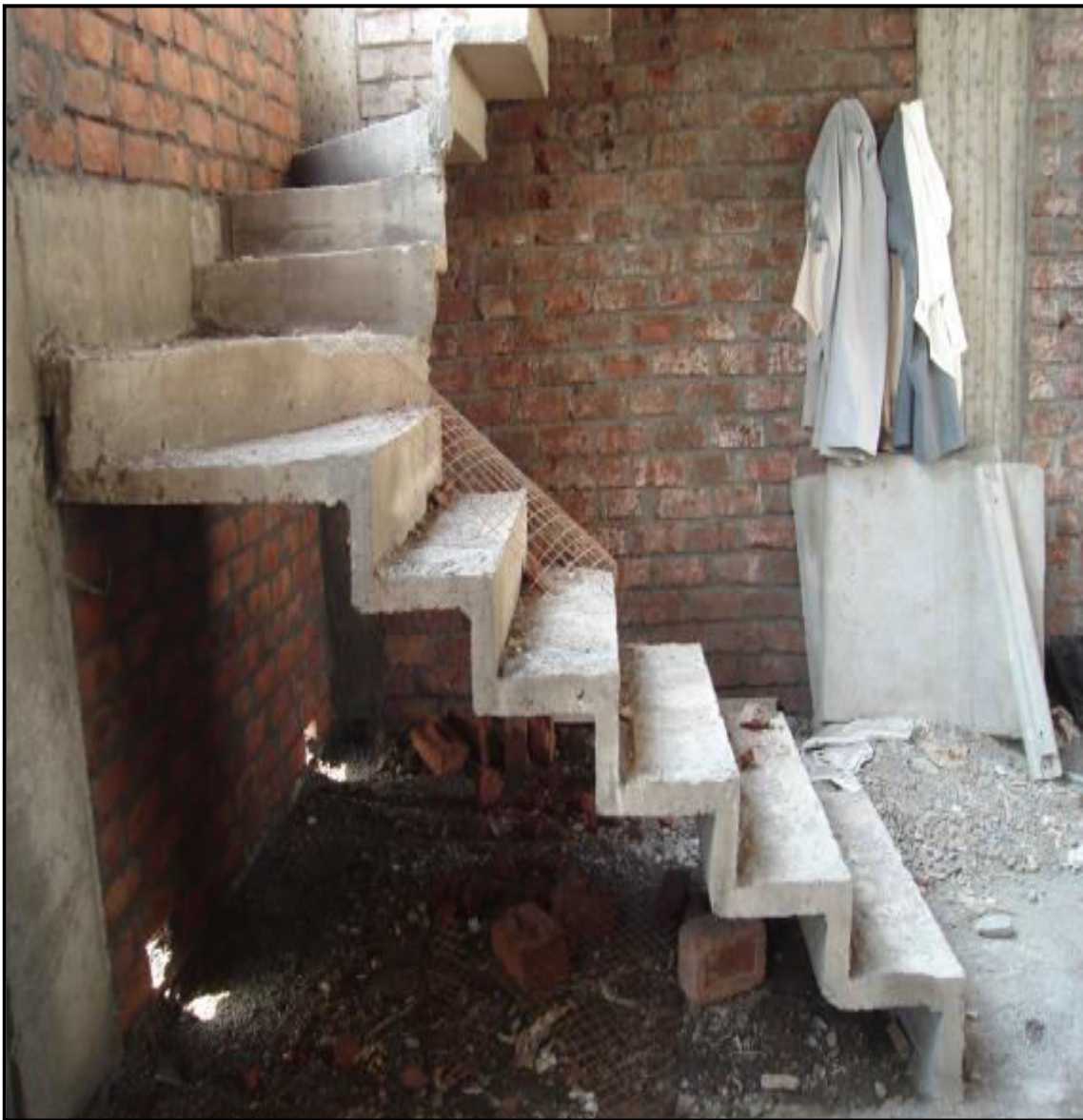
Typical Ferrocement Staircases.
