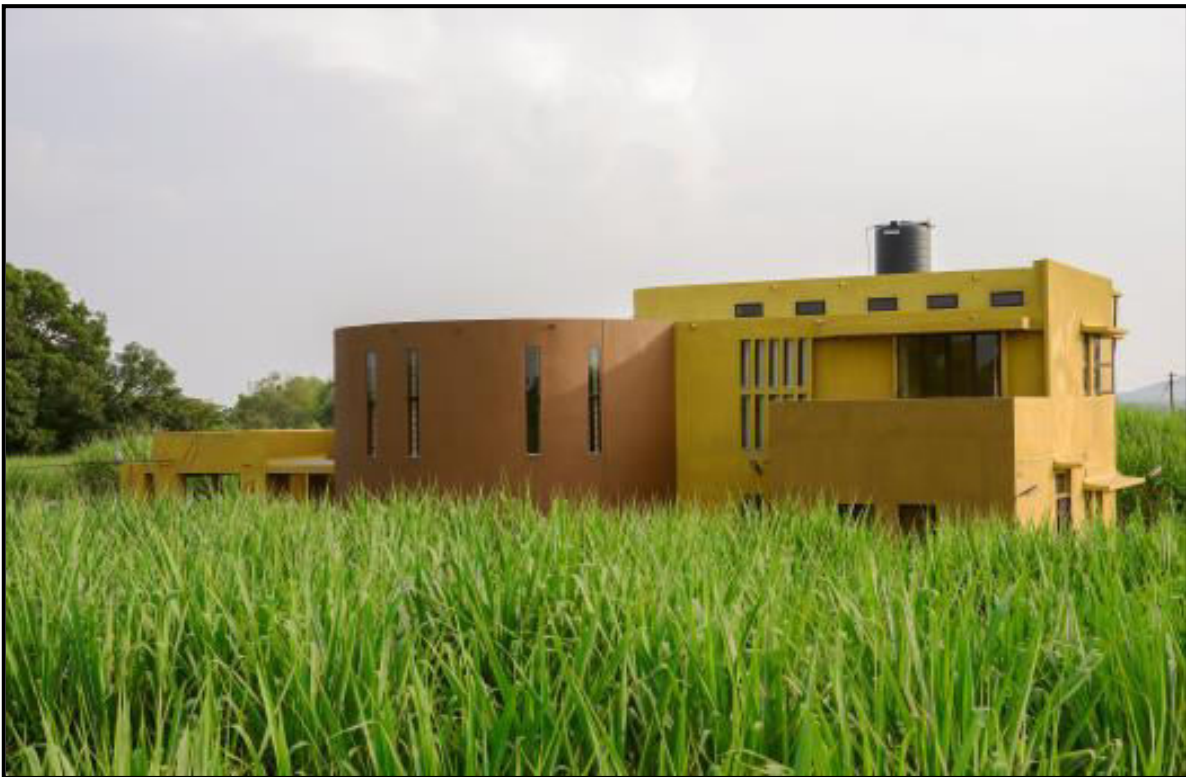
Ferrocement house built in Village Gove, Dist.Satara, Maharashtra.
