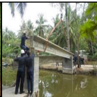
Fixing of 30 feet ferrocement precast bridge
