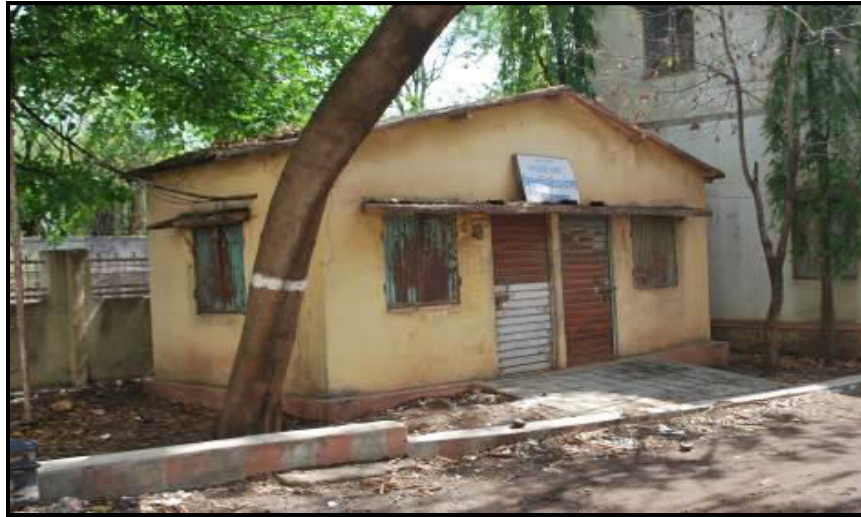
Fig 7.36 A building for wireless system at Osmanabad Irrigation Colony, built under the Chief Engineer, WRD. in 1995. (Still in tact)
