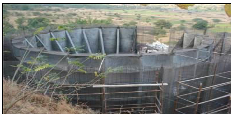
Fig 7.26 Water tank near Talegaon Dabhade, Dist Pune.
