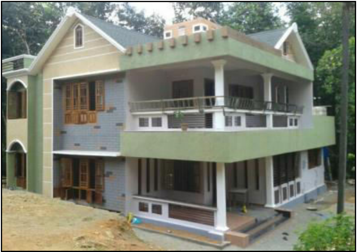
Ferrocement House built in Chenganasserry, Kerala.
