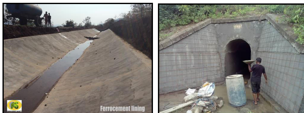
Fig 8.6 Ferrocement canal lining at Kalwan, District Nashik in 2014
