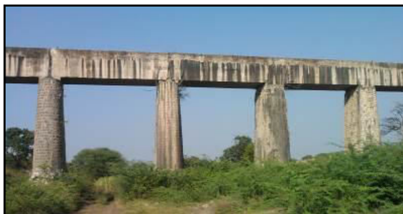
Fig 7.32 Jacketing the abutments and piers
