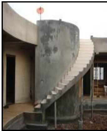
Fig 7.5 Steps using ferro-cement built near Katraj, Pune
