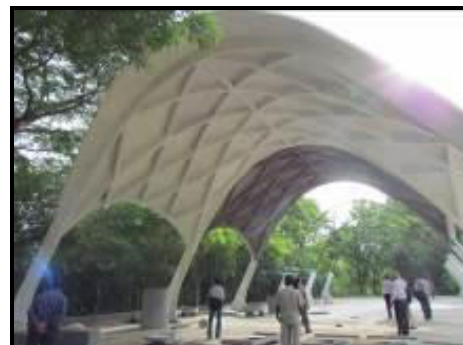
A motor shed built in ferrocement at Auroville, Podicherry.
