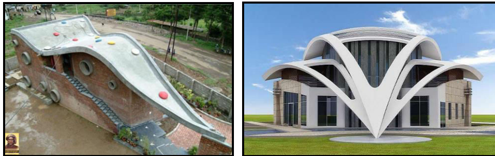
Fig 8.8 Space structure in ferrocement-2
