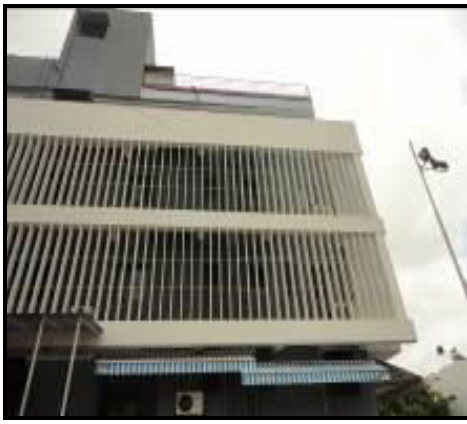
Fig 7.3 Ferro-cement fins at Satara Hospital
