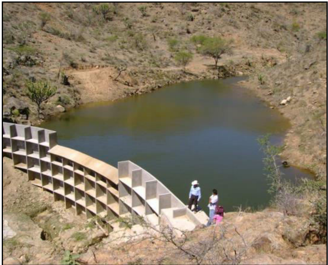
Ferrocement dam in Mexico
