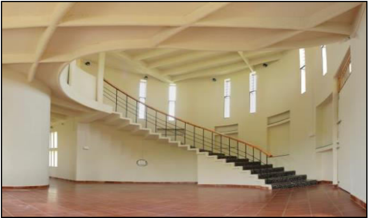
Ferrocement house built in Village Gove, Dist.Satara, Maharashtra.
