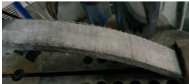
Figure 10. Crack on the top face of arch
