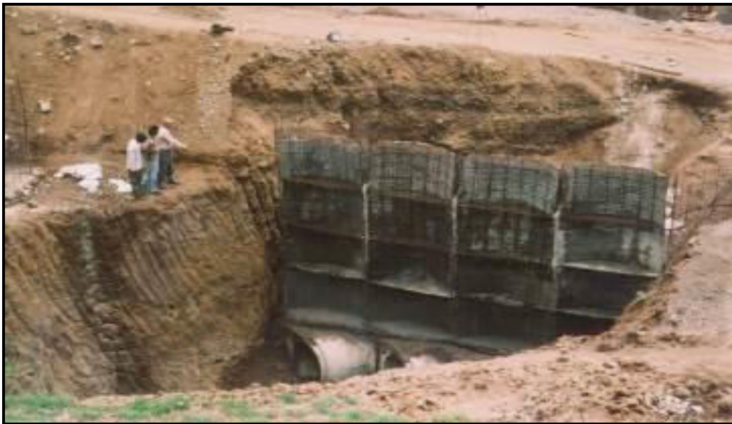
Fig 7.16 Ferrocement counterfort retaining wall
