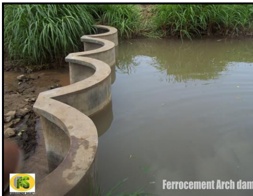
Fig 8.11 Dams at Pune, India
