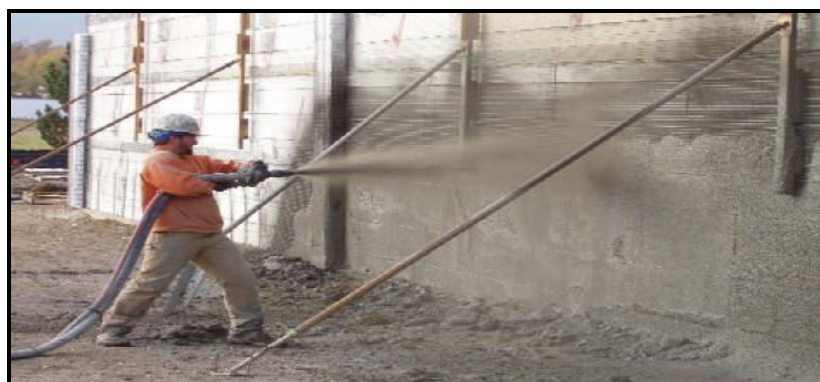
Fig. 4.6 Guniting machine and nozzle
