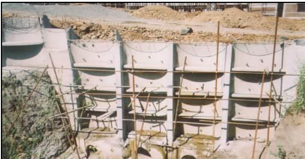
Fig 7.15 Ferrocement retaining wall
