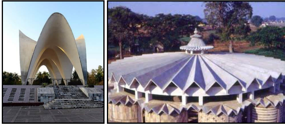
Fig 8.7 Space structure in ferrocement-1
