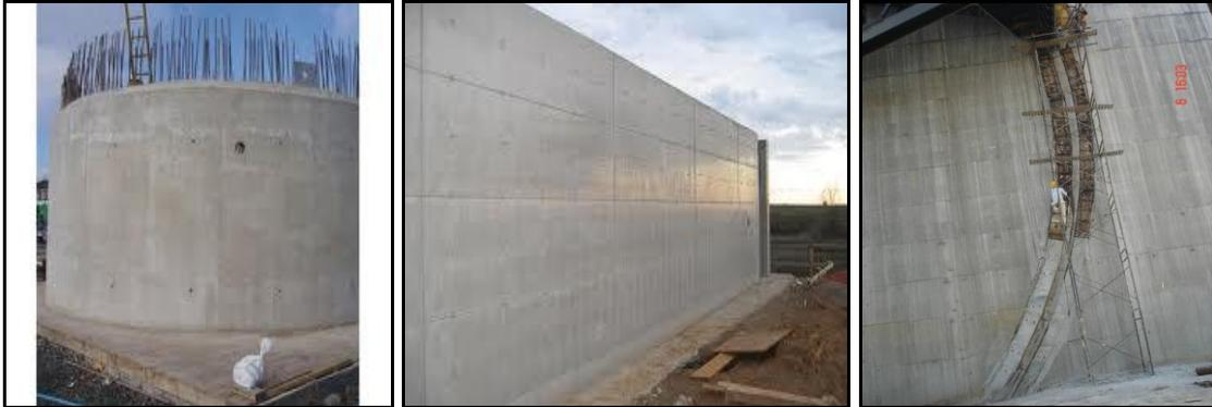
**Photograph 9. Photos showing finished surface of SCC**
