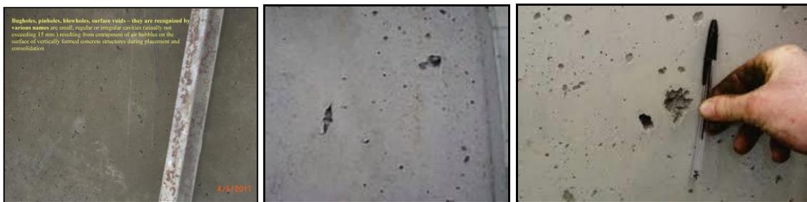
**Photograph 10. Photos showing the bugholes on concrete surface.**
