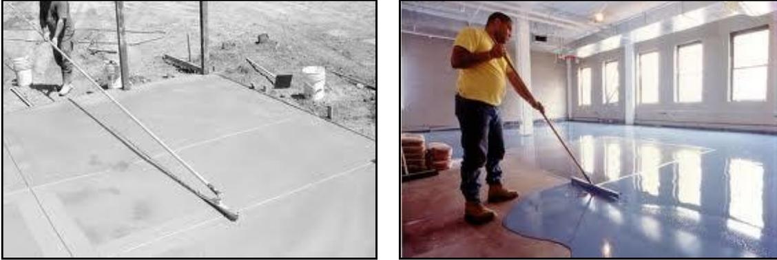
**Photograph 8. Leveling SCC with a skip float**
