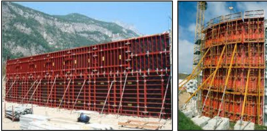
**Photograph 4 Formwork erected for SCC**
