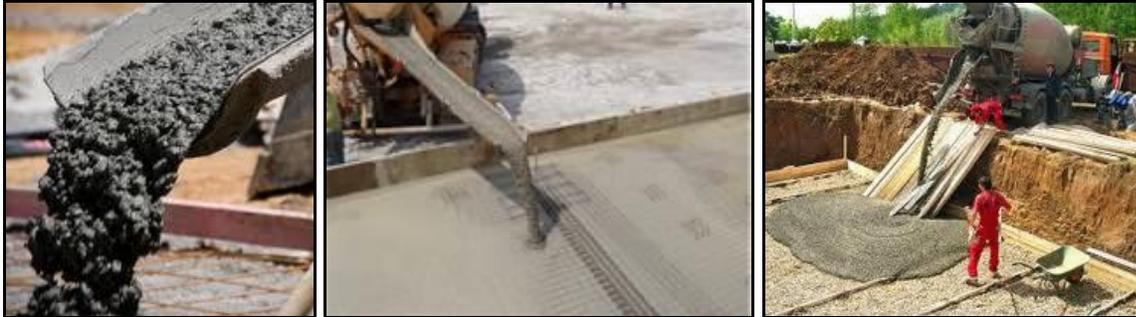
**Photograph 6. Photos showing SCC discharging through truck via chute**
