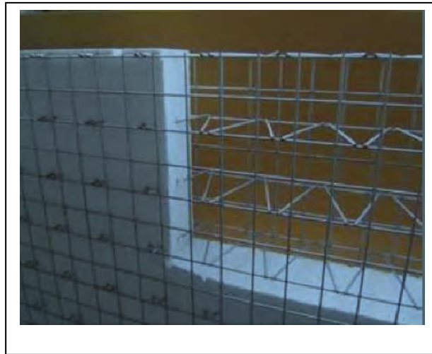
Fig 2: Reinforcing mesh expanded polystyrene core and diagonal wire.
