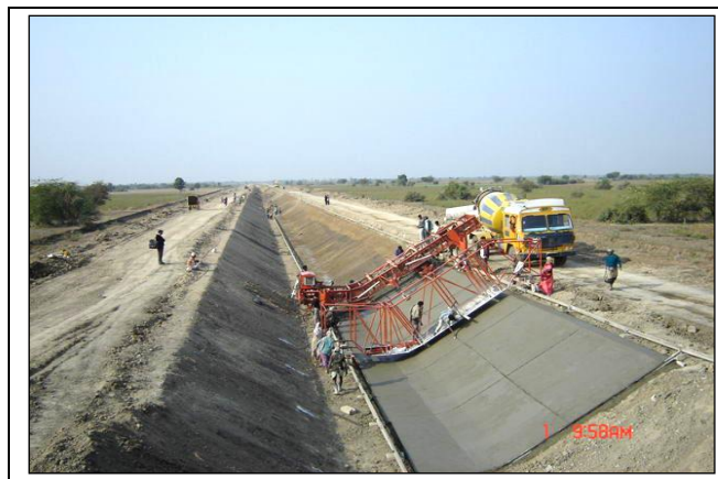
Photograph 6 (h): Canal Lining Using Paver
