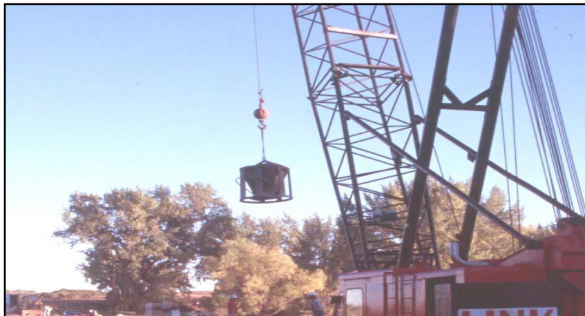
Photograph 6 (a): Placing Concrete with a bucket
