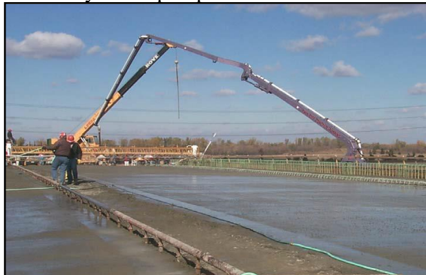
Photograph 6 (d): Concrete placement by a boom pump
