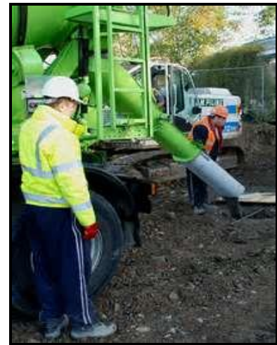
Photograph 11: Placement of concrete by pump
