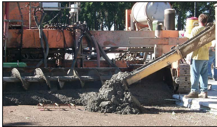
Photograph 6 (b): Placing concrete from the end of a chute
