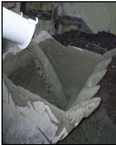
Photograph 11: Placement of concrete by pump
