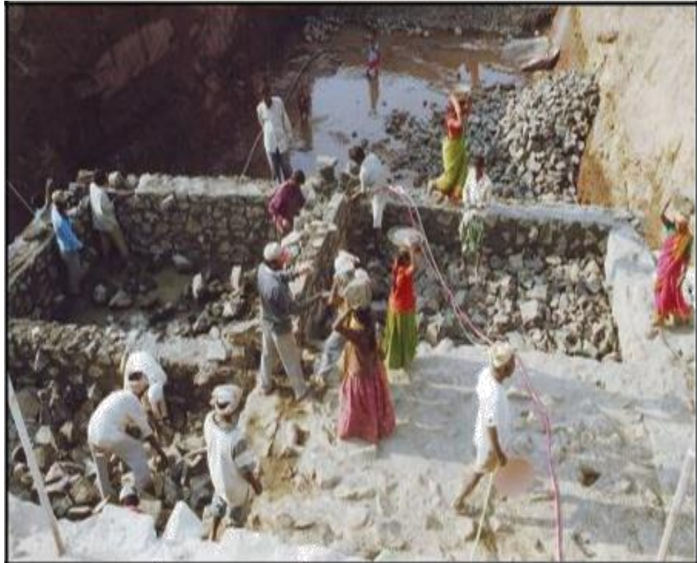
Photo no. 4: Laying of stones in compartment
