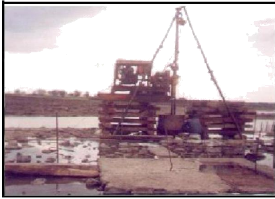
Photo no. 6 : Drilling core by drilling machine at site
