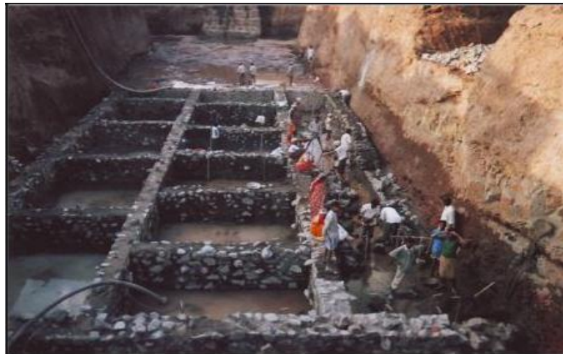
Photo no. 3 : Partition wall compartments for construction of colgrout masonry
