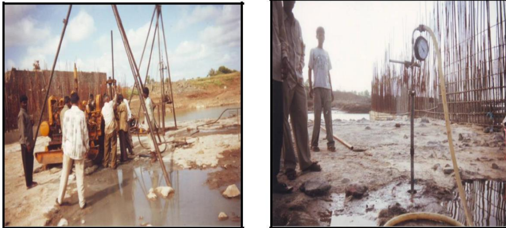
Photo no. 5 : Drilling of hole and testing for in-situ permeability
