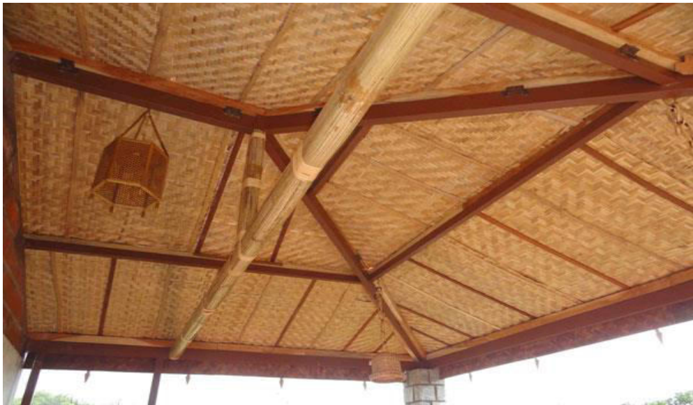
Bamboo used in roof
