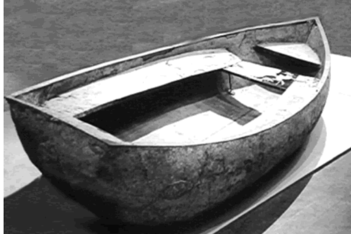
Fig.no.1-First boat of Ferrocement constructed by Mr.J.L.Lambot
