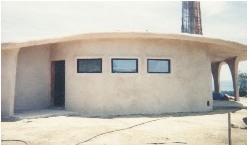
Fig. No.16- A typical ferrocement house
